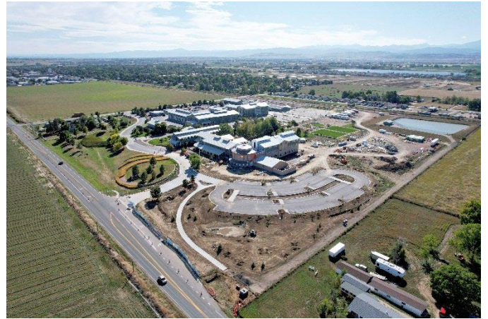
An aerial view of the Northern Water Berthoud headquarters in 2023.
